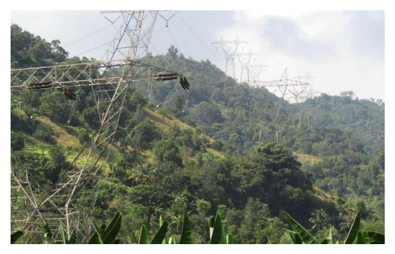
With the support of contractors KSO PT Sangkan Jaya and PT Prima Estika, PLN (Persero) TJBB completed and energized their 500 kV quad bundled Suralaya to Balaraja transmission line on December 30, 2019. The project started on November 12 and was completed very quickly by using six separate teams on six defined sections. Support for the installation was also provided by PLN, PLN Engineering, PT KMI Wire and Cable Tbk, and CTC Global's Licensed Service Provider PT Dinamika Elektra Mandiri.
